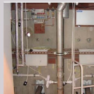
Prefabrication reduces on-site labour and instal time
