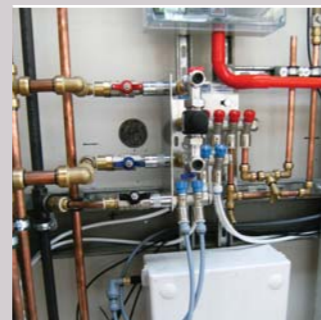
TMV Manifold with double check valves ...
